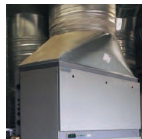
Wall-mounted dehumidification system
